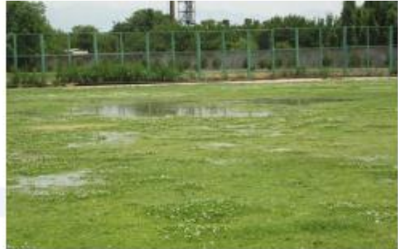
Poor surface levels, poor drainage and weed invasion
