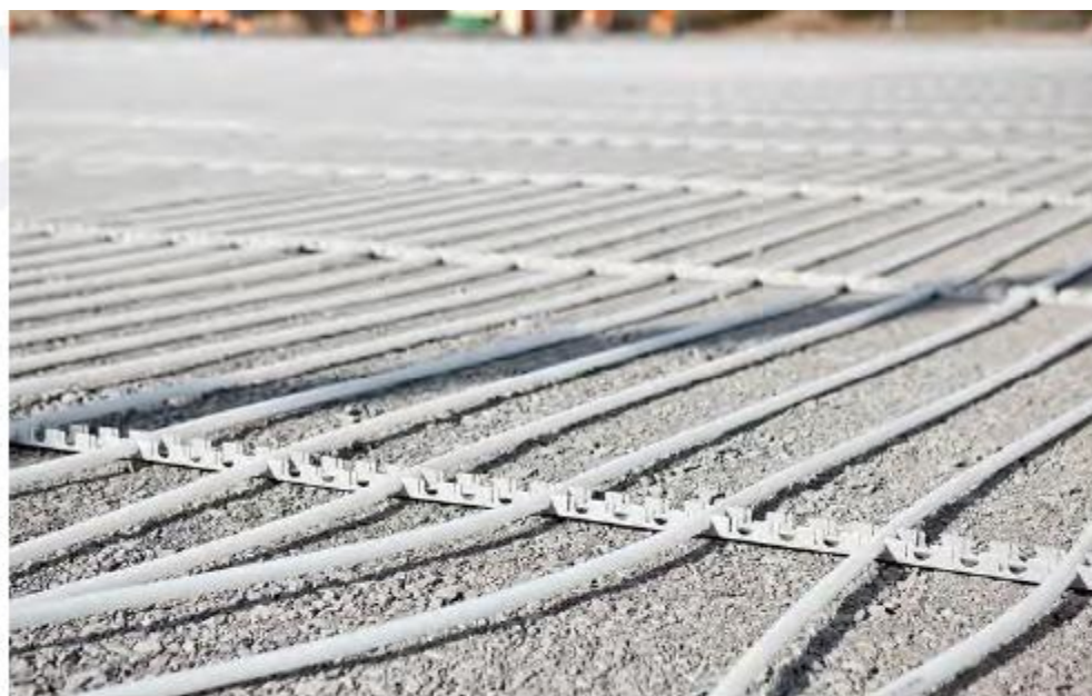
Figure 11: Pipe heating system installed in holding racks on the gravel drainage layer to support the pipes prior to root-zone installation
