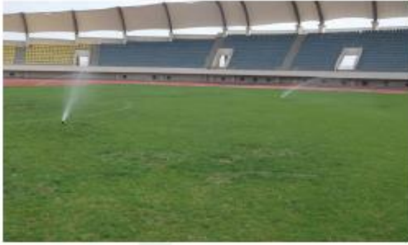
Irrigation system with poor coverage due to the sprinkler overlap arrangement
